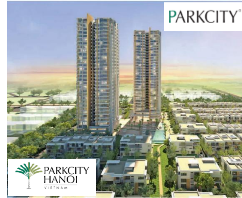
PARK CITY RESIDENCE – HA NOI (Vietnam) 2022
