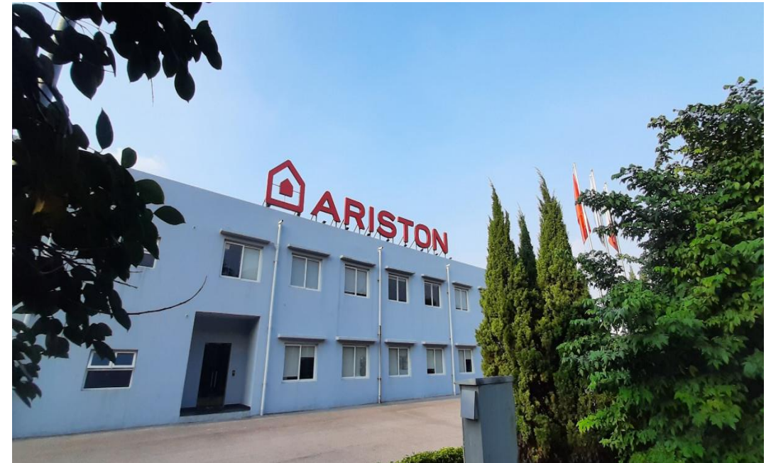
ARISTO FACTORY – BAC NINH (Vietnam)
